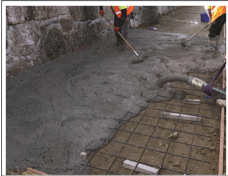
Figure 4 BFRP Rebar installation on site
